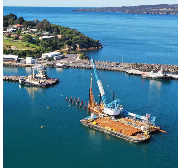
Figure 4: Pile installation of the Eden Attenuator using a jack-up barge.
